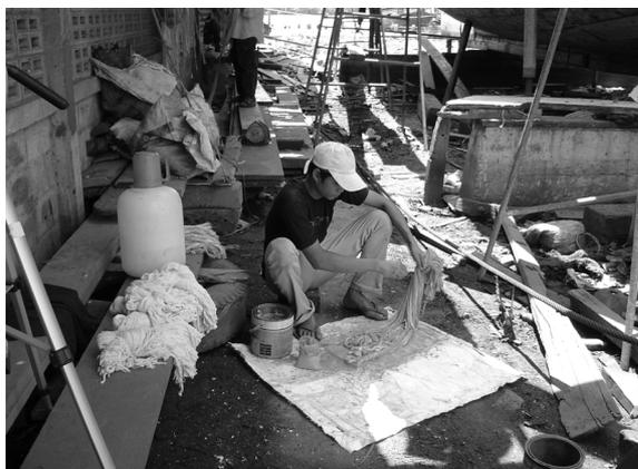
Fig. 1. Mingling lead oxide and yang oil with cotton yarn.
